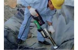
Thanks to its length, the FUSION 3 is particularly suitable for civil engineering applications.
