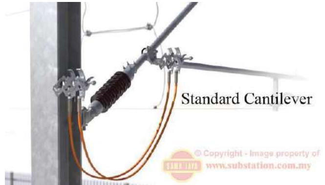
Cantilever Section using Double Short Rail Earth
