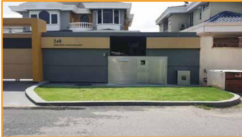
*Laser Cut Address & Stainless Steel Meter Box Cladding*
