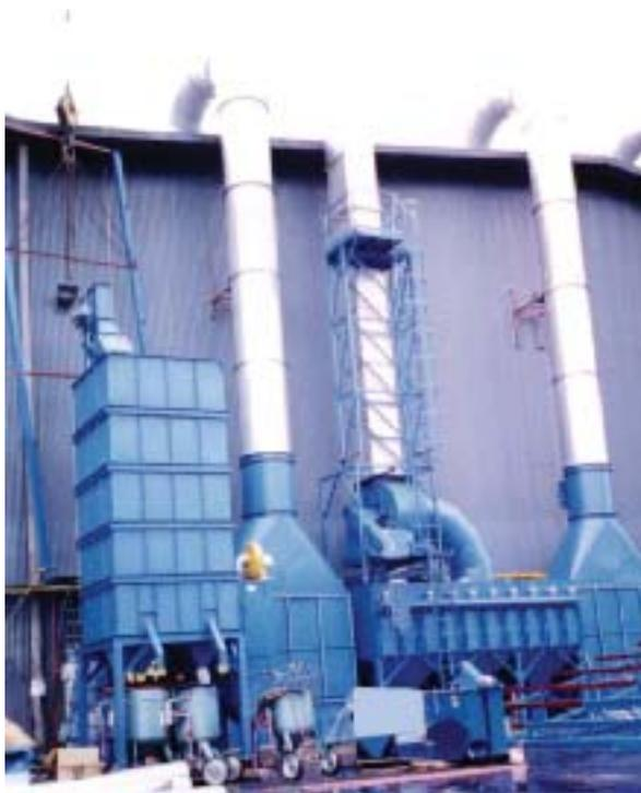
**Dust Collectors** are used for removal of blasting dust. It also serves to maintain a designated number of fresh air changes inside the room. A room of size between 850m<sup>3</sup> to 2800 m<sup>3</sup> is recommended to use an air change of every five minutes.
