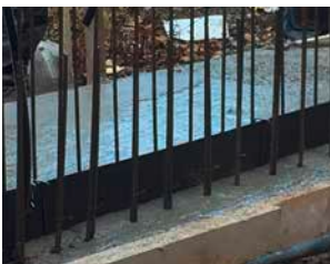
AQUAFIN-CJ5 when installed.
