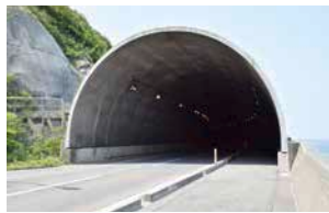
Tunnels and concrete pipes
