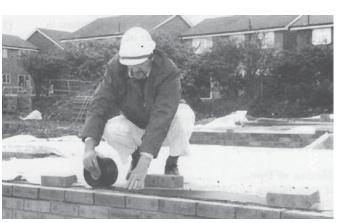
**Brickgrip** is a flexible Damp Proof Course membrane (DPC) manufactured specially for use in bricks, cement & sand blocks, stone works and concrete walls of either solid or cavity wall construction. It is suitable for use in horizontal or in stepped positions and is compatible with all materials with which it is likely to be in contact with in normal construction.
