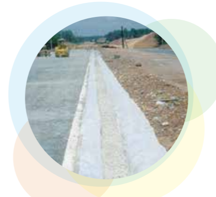
Standard Geotextiles used in a French Drain application.
