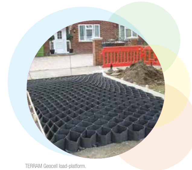
TERRAM Geocell load-platform.
