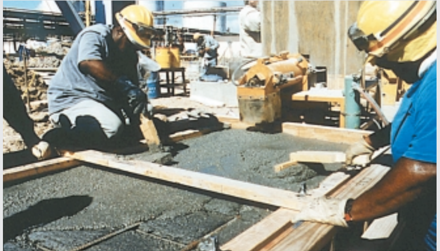
Polymer concrete is easy to install and negates the vulnerability of surface defects.
