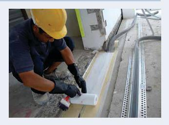
MIGULINE is used in association with BONDER A2 where Expansion Joint treatment is made.
