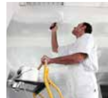
Renovation Works - Home Central Air Conditioning Commissioning
