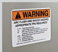
Arc Flash Labeling
