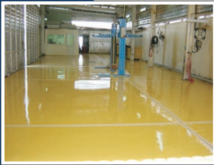
Teyseer Center Auto Workshop- Qatar
