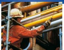
Excellent adhesion and wetting properties mean small areas can be touched up either on intact primer, whatever the type, over other topcoats in good condition or direct to metal (150µm) will give light corrosion protection (class C3).
