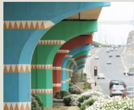
Abha Bridge, Abha, KSA
