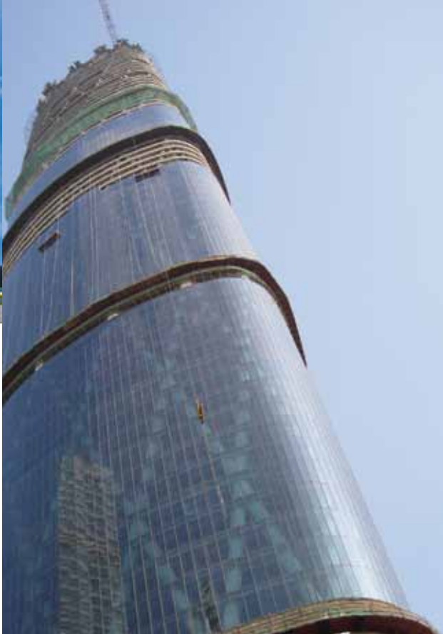
Jotun coating systems protect Guangzhou West Tower, Guangzhou, China
