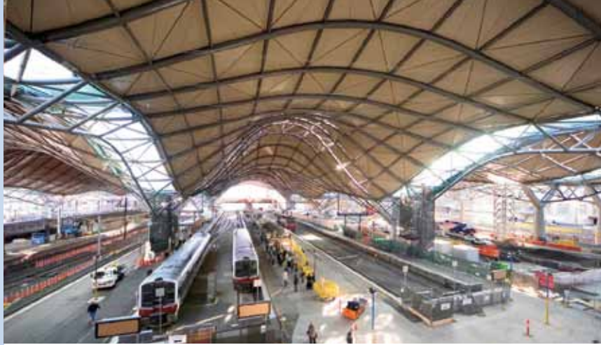
Jotun coating systems protect the US$600m Southern Cross Railway Station development in Melbourne, Australia.
