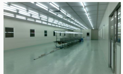
CLASS 1000 CLEAN ROOM
