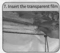
7.Insert the transparent film to the lower back of the air conditioner.
