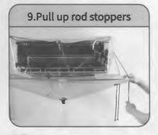
9. Finally pull up rope stoppers around the four corners to the same level to finish the installation.
