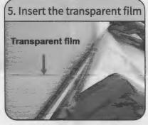
5.Insert the big size of transparent film in the back of the air conditioner and tighten the cleaning cover by adjust the rope stopper.
