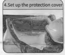
4. Place the protection type cleaning cover on C shaped support bracket, insert those two small transparent films on both side in the back of the air conditioner.
