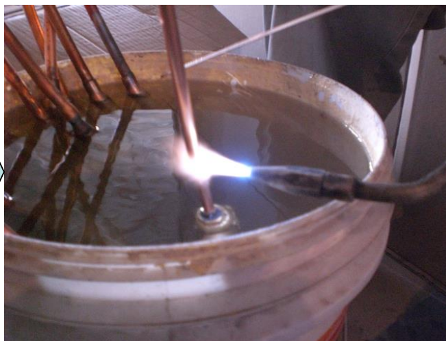
Brazing work is performed
