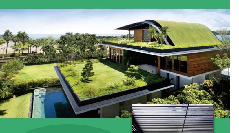
A green roof system is the roof of a building that is partially or completely covered with vegetation and a growing medium planted over a waterproofing membrane. It may also include additional layers such as a root barrier and drainage and irrigation systems. PENTENS T-100 is a water based polyurethane membrane which is suitable for green roof system with its high elongation that can improve waterproofing performance.
