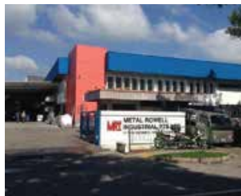
Aluminium Fabrication Factory
