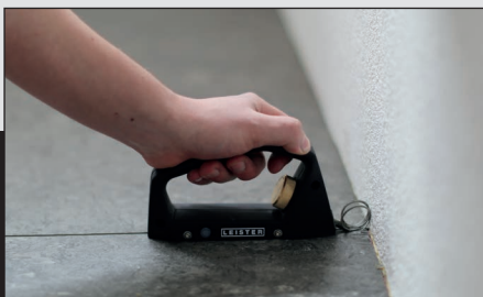
Executing clean grooves up to connecting walls
