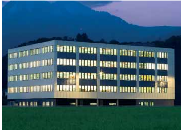
Headquarters in Sarnen, Switzerland
