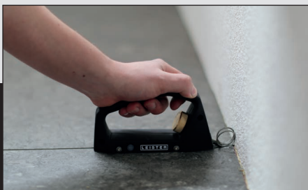
Executing clean grooves up to connecting walls
