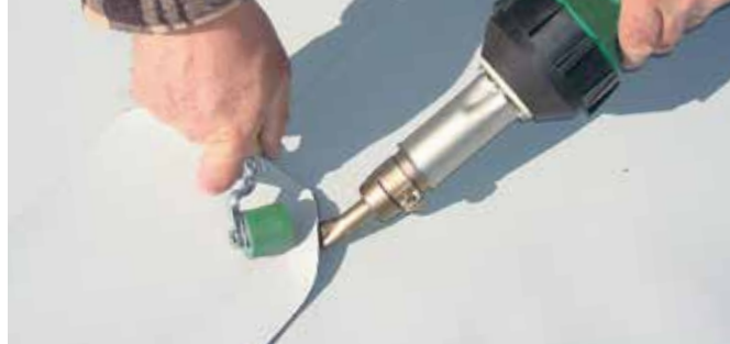
TRIAC S while overlap welding on the roof.
