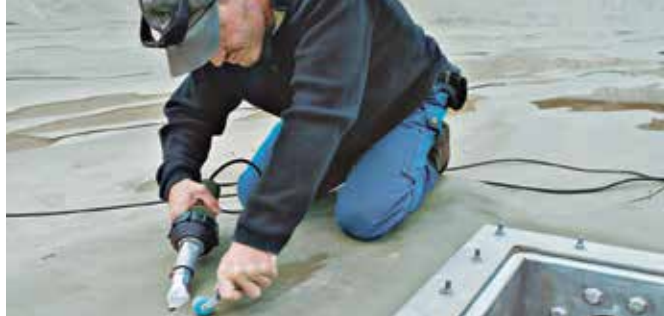
TRIAC S in use welding a future a storage reservoir.
