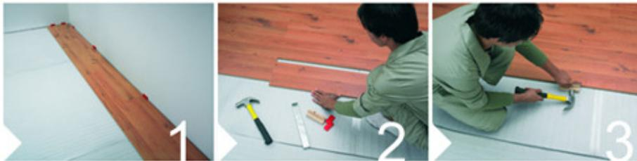
**8. In case the wall is so incline, please keep space from wall. By the narrowest point must have 30 mm space from wall and the broadest area must not over 18.5 mm.**
