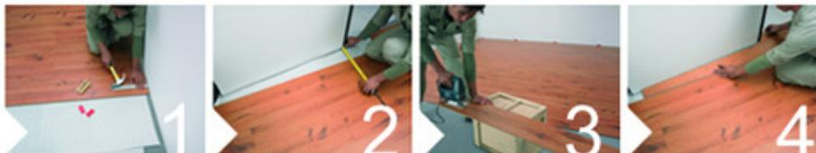
**10. Paving floor until the end of room, the last line must deduct 10 mm from total space of last line to wall. Then, cut the size to fill all area and put bars to fit every point.**
