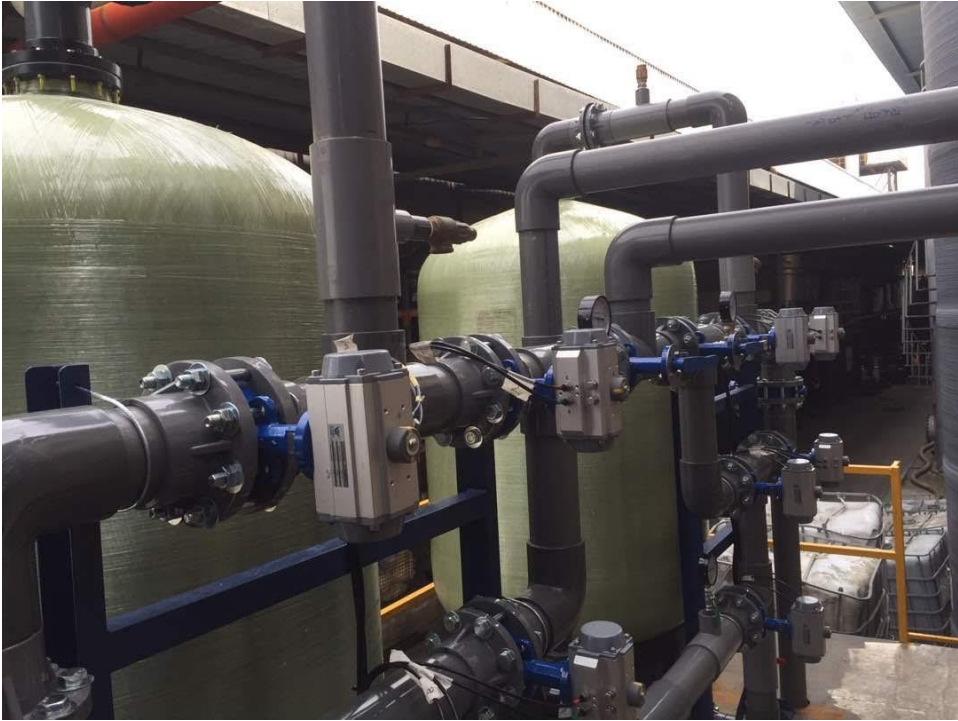
Auto Media Filter - Pneumatic Actuator Valves
