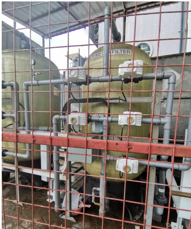
Auto Media Filter – Motorized Actuator Valves
