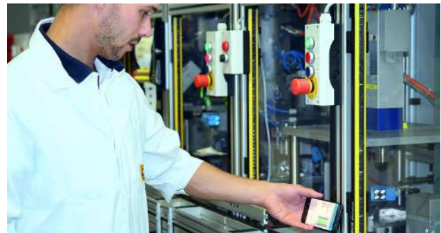
Figure 7: Safeguarding of a machine and diagnostics on the protective device
