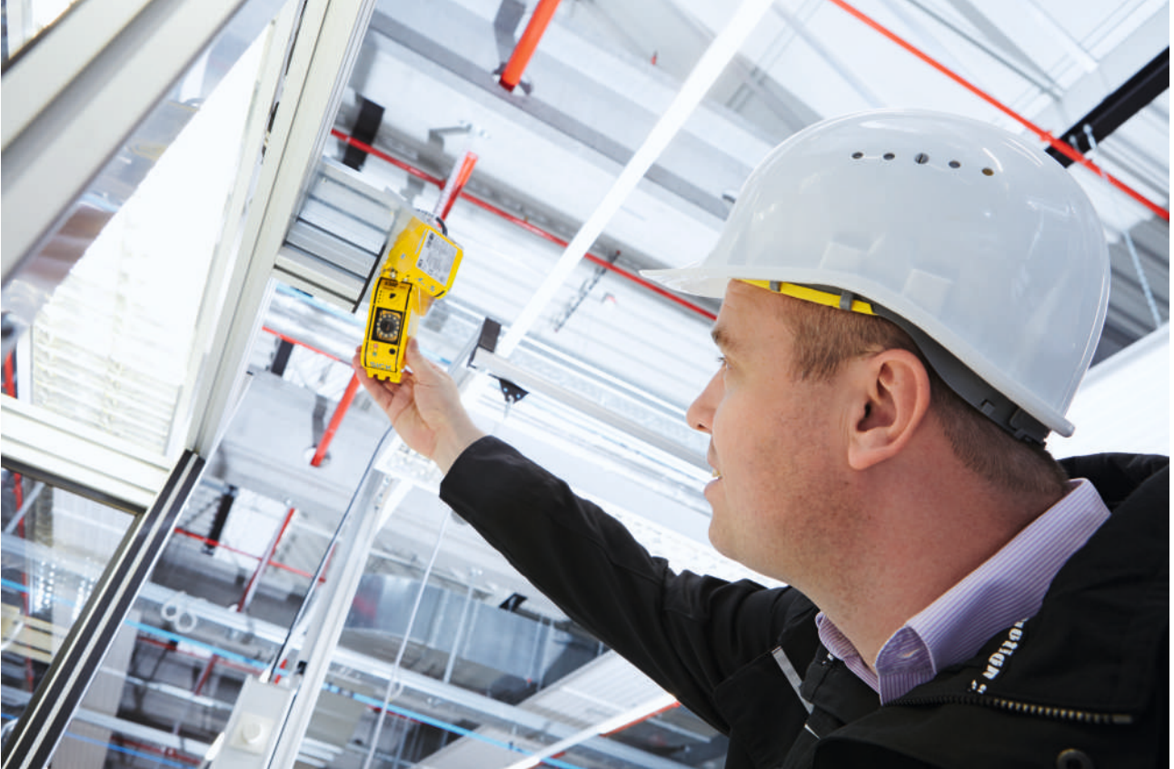
Figure 119: Service employee inspecting a protective device
