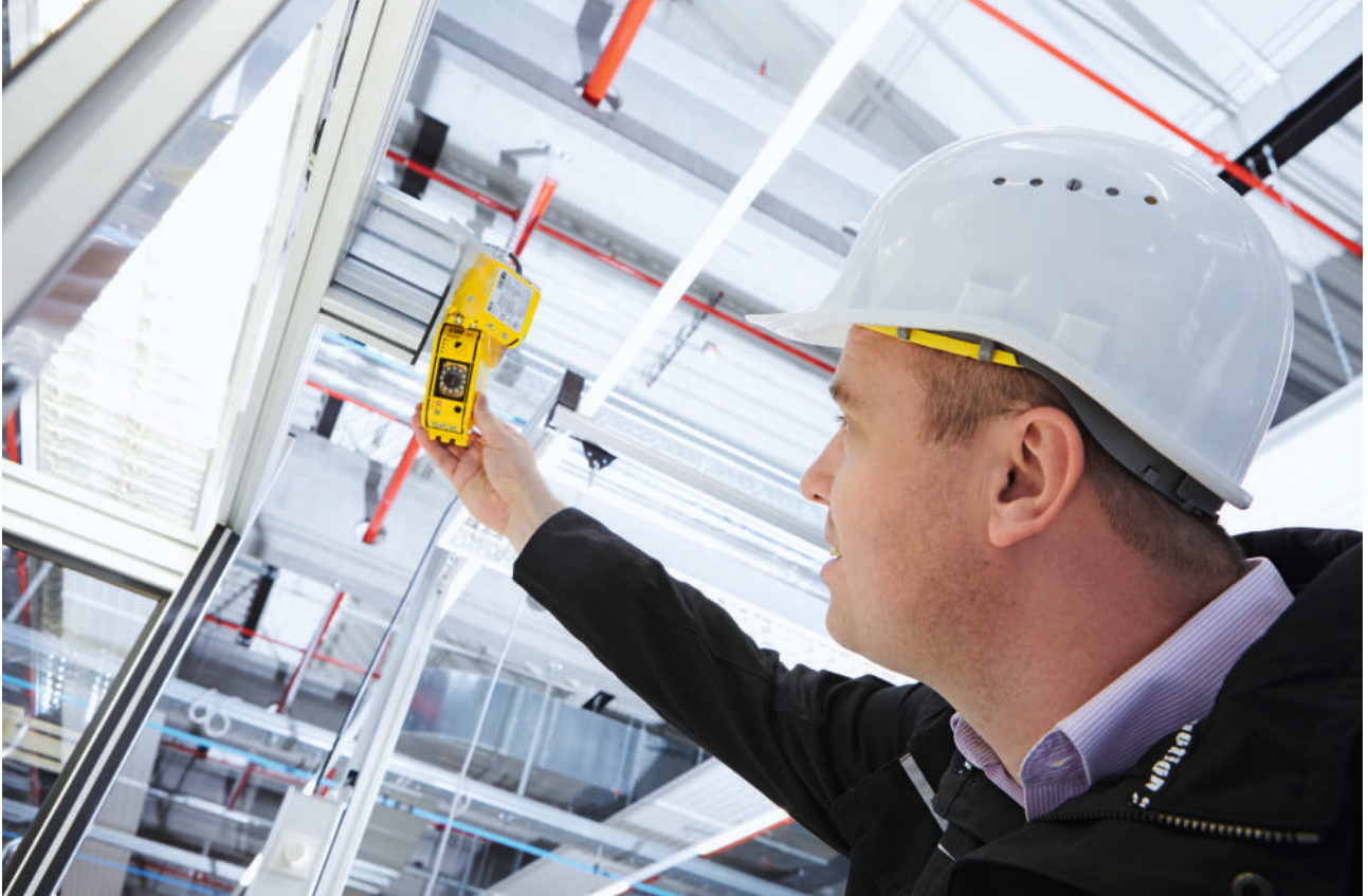
Figure 119: Service employee inspecting a protective device
