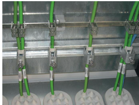
Figure 8: Large-area connection of the shielding to ground busbars
