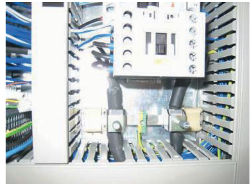
Figure 8: Large-area connection of the shielding to ground busbars
