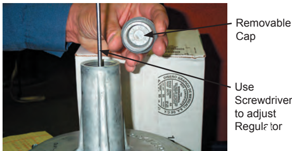
Figure E-9 Main Gas Pressure Regulator Adjustment
