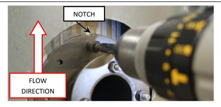
Figure 8: Fastening the First #12 Sheet Metal Screw
