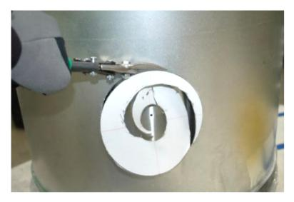
Figure 5: Shearing 6" Hole with Aviation Snips
