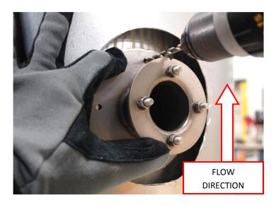
Figure 7: Collector Orientation & Marking the Top Hole
