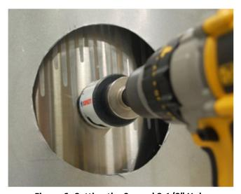
Figure 6: Cutting the Second 2-1/8" Hole
