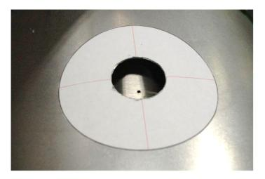
Figure 4: Result after Cutting the 2-1/8" Hole
