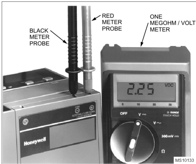
Fig. 11. Measuring voltage flame Signal with 7800 SERIES controls
