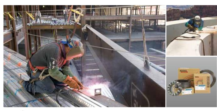
Innershield® NR233 is a good choice for training or novice welders while also meeting the mechanical property requirements listed in AWS D1.8. It is recommended for vertical up and overhead fillet and groove welds. This wire is easy to use and has high deposition rates making it a "win-win" wire for many applications. For easy out-of-position operability and impact properties capable of exceeding 27 J at -29°C – choose Innershield® NR233.
