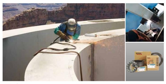
Innershield<sup>®</sup> NR-311 is designed for the welding with high deposition rates and fast travel speed. It is recommended for fillet, lap, and butt welds on 3.2 mm (1/8 in.) and thicker steel, including some low alloy steels in applications without impact strength requirements. It's also a good choice for crack resistant welding on high sulphur steels.
