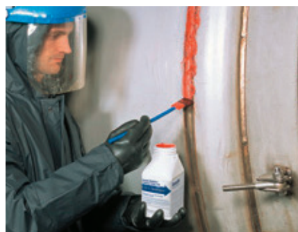
Photos showing the application of RedOne™ Pickling Paste and pickling at low temperature (+8 °C) of high alloyed heat exchanger 2205 (1.4462)
