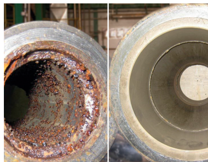
Photo: Result with Bath 302 before and after circulation pickling
