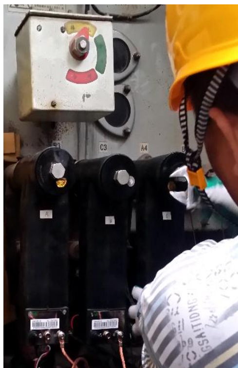
Figure 5 RMU Type HV Energy Meter Installation Method
