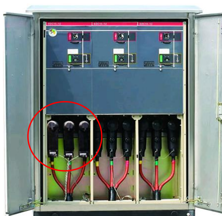
Figure 7 HV Energy Meter Solution (Cable Accessories Plug in Type Installation)
