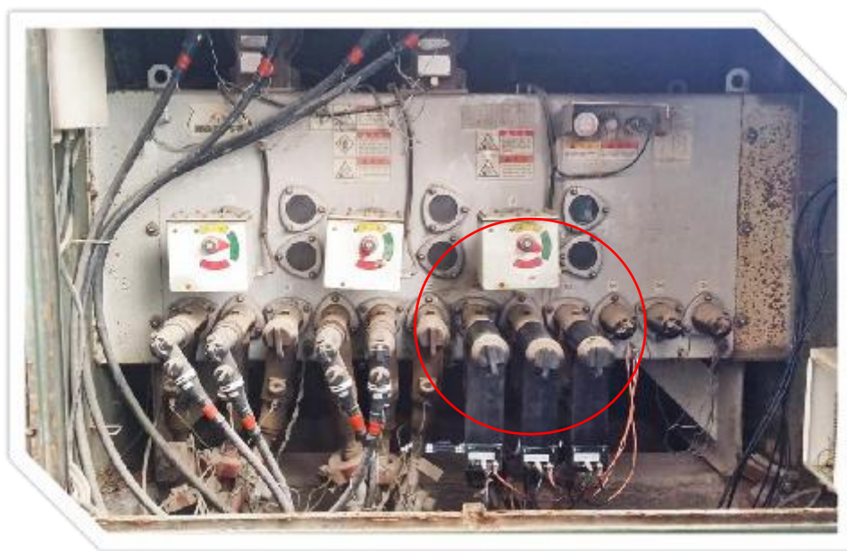
Figure 1 RMU Type HV Energy Meter Installation Example
