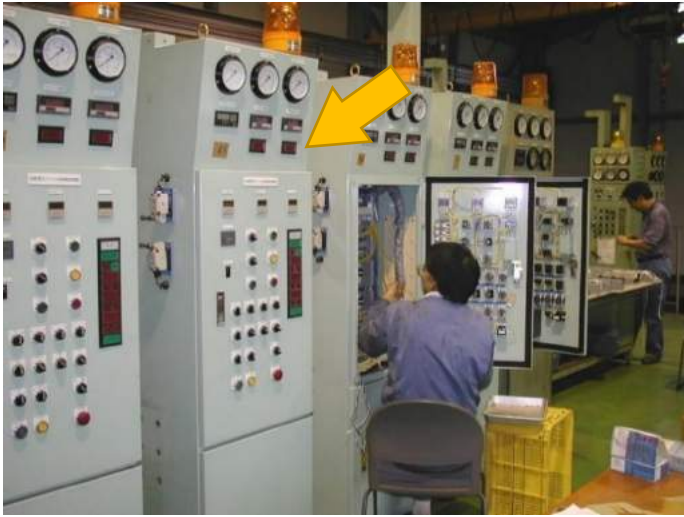
1) There are so many control panel in most of factories. Also you can see digital panel meters on the surface of panel.
