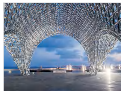
Heavy Steel Structure
