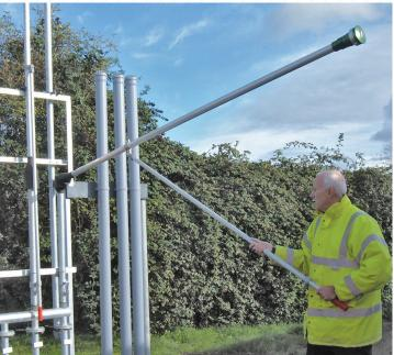
Easy to retro fit to existing vent systems no cherry pickers, scaffolding or step ladders – swivels your vent riser to working height for easy access to change valves
