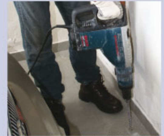
Concrete slabs have to be drilled.
