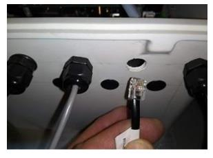
Carefully insert the connectors thru treaded holes at bottom of control panel.
