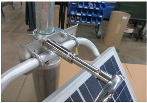
Attach solar panel (if equipped) with saddle brackets and face flat side of bracket to the South and raise panel at appropriate angle to maximise angle with sun depending on time of year. Make sure this bracket is high enough on the upper mast section to allow room for the control panel to be mounted next.
