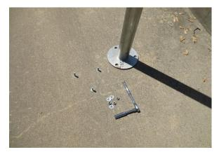
Anchor your mast base onto a flat and level concrete pad, see attached hole layout
