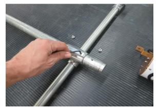
Slip the cross-arm tube assembly on the 1.25" upper mast section. Center it between the 2 holes where the rain gauge bracket attaches if purchased.
