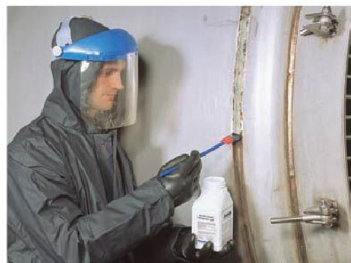
Avesta Classic Pickling Gel 122 - easy to apply thanks to its free-flowing consistency.
