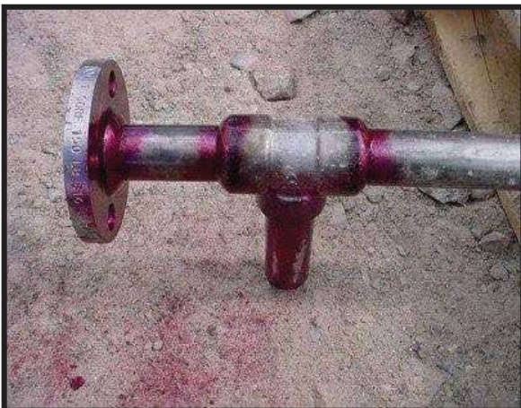
“ Pipe Joint Dye Penetrant Inspection ”
