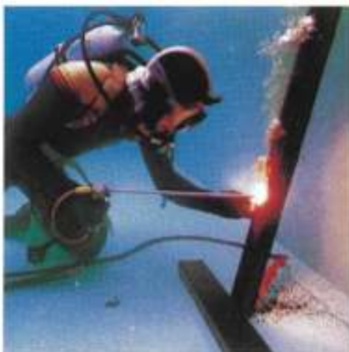
Under water cutting 水中切断
