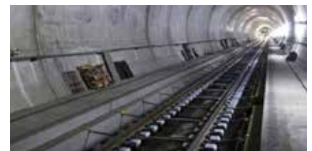
UNDERGROUND TUNNEL JOINT
