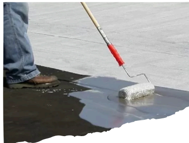
RE-COATING (OLD & NEW) WATERPROOFING
