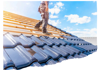
RECTIFYING ROOF TILES
