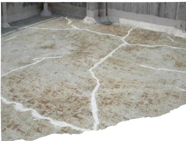
SEAL CRACK & JOINT
