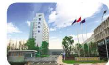
University and Quality inspection institute
