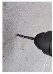
10. Drill 4 holes for racks base (Recommend make a marking by rack base first, before drill)
