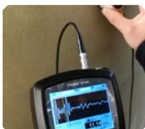
FRP Oil Tank
